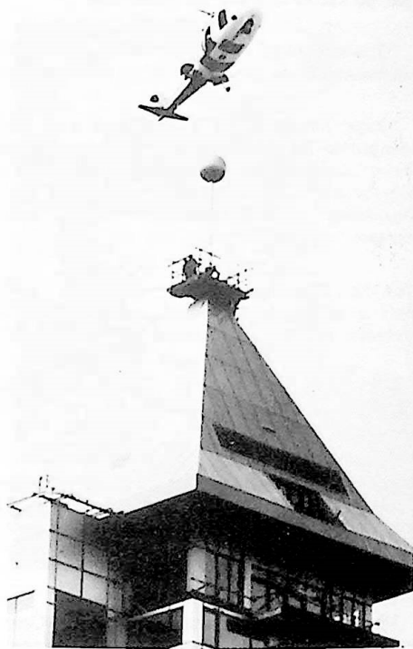
Helicopter lift held while the new tidal ball is fixed onto the apex of the Belvedere Tower where it will act as a tidal indicator at the new Chelsea Harbour development.
