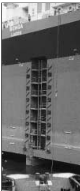
Pilot boarding point
